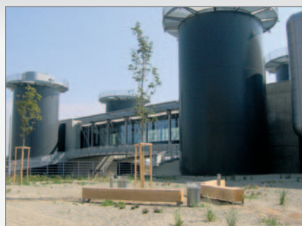
08/2007 Connecting bridge and power plant towers
