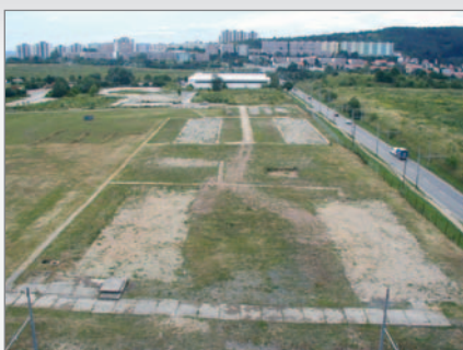
08/2004 The Bohunice site before construction began
