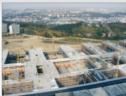
03/2006 The Blue Stage under construction
